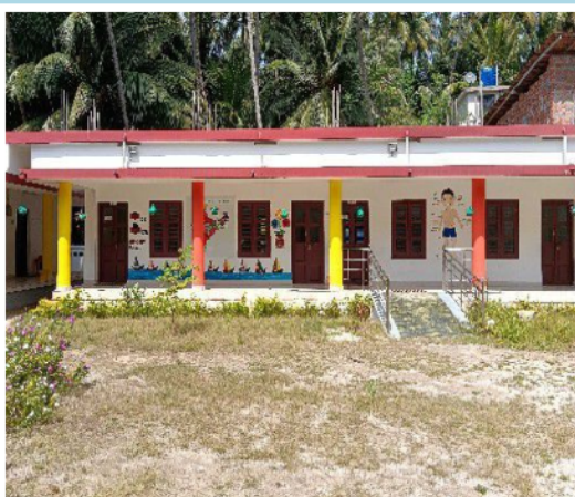
Polling Station Building Front View
