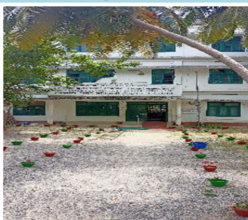
Polling Station Front View
