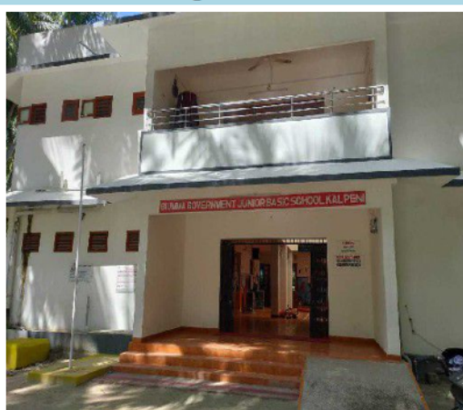
Polling Station Front View
