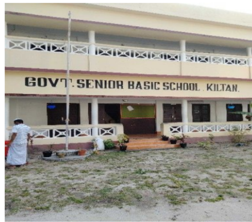
Polling Station Front View
